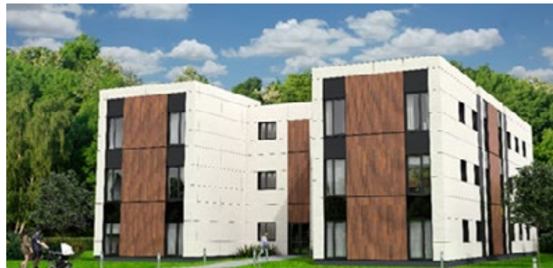
Gas Works site, Grangetown - new supported accommodation for families.
