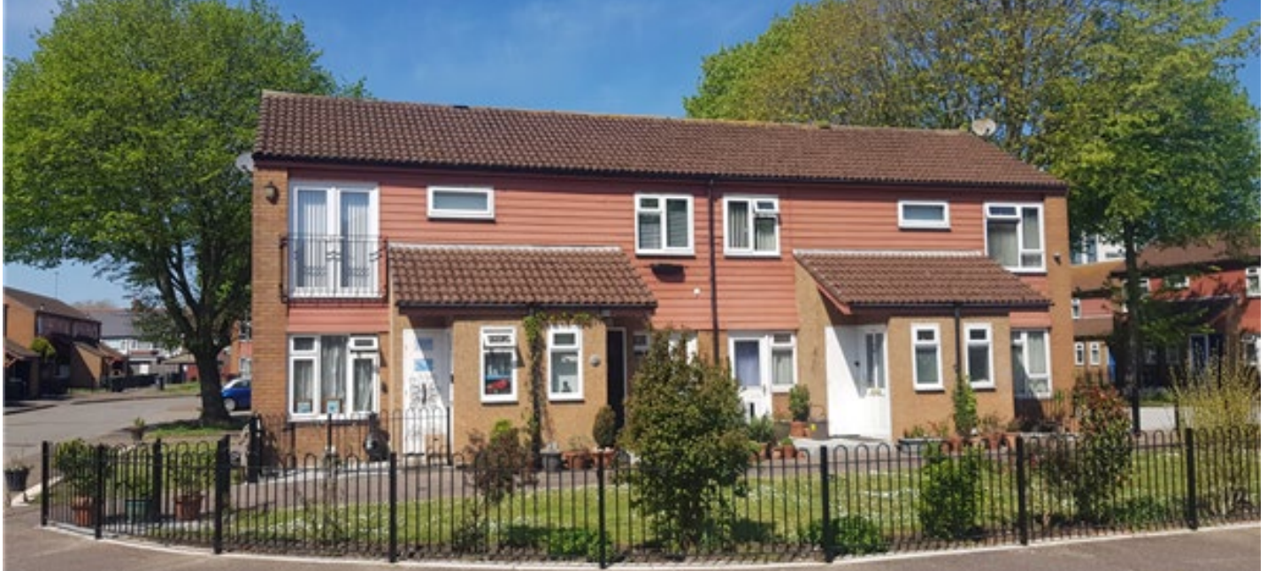
Regeneration works to Taff embankment
